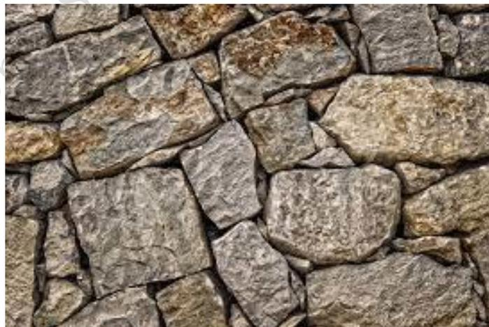
Fig 1.1 Rubble Masonry
