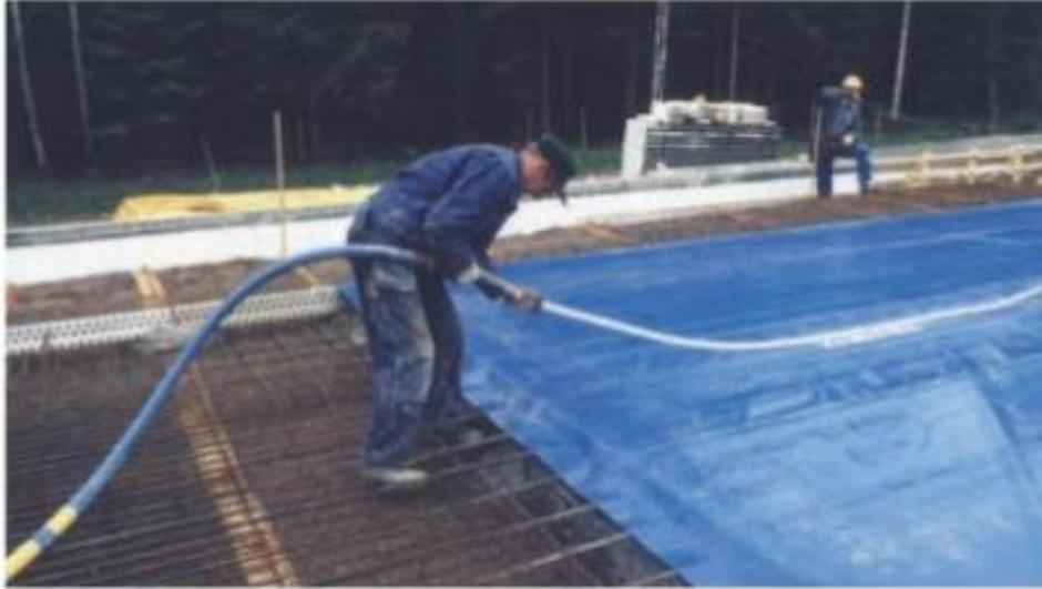
Fig 2.12 Top cover is connected to the suction of the vacuum pump. It is important to check that top cover seals against the fresh concrete outside the filter pads
