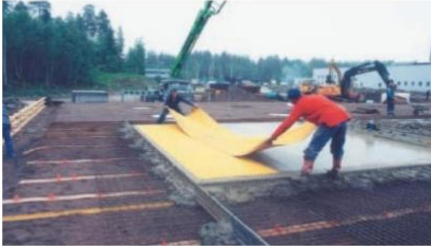
Fig 2.10 Filter pads are placed so that there will be a sealing edge around the entire filter pad surface
