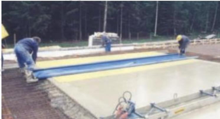
Fig 2.11 Top Cover is unrolled over filter pads
