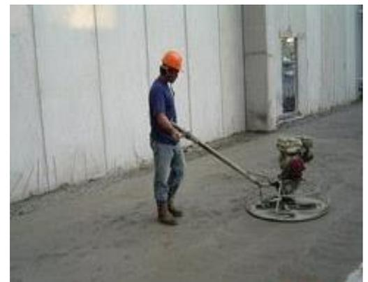
Fig 2.6 Using Floater Machine
